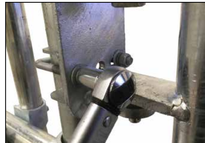
E. Torque all nuts/U Bolts to 39Nm using the 13mm or 17mm socket and torque wrench. Repeat steps A-D for right hand side gate.
